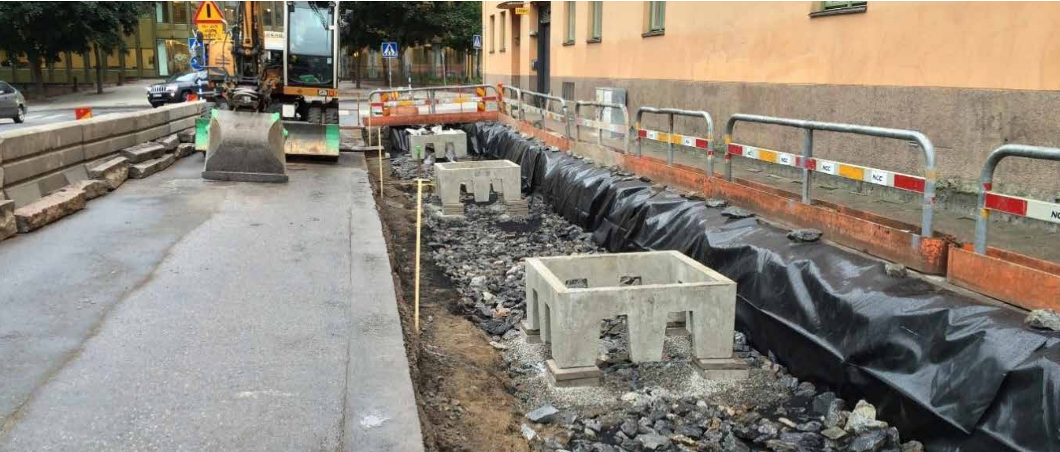
Reference: Hellman, F. et al. (2012). Draining hard packed surfaces in a city environment – breakdown tests with HVS equipment at VTI. Statens Väg-och transportforskningsinstitut (VTI), Sweden. Figure 13: A structural soil tree pit in the process of construction. In this instance larger aggregate is being used so that the final surface will be able to support heavy traffic.
