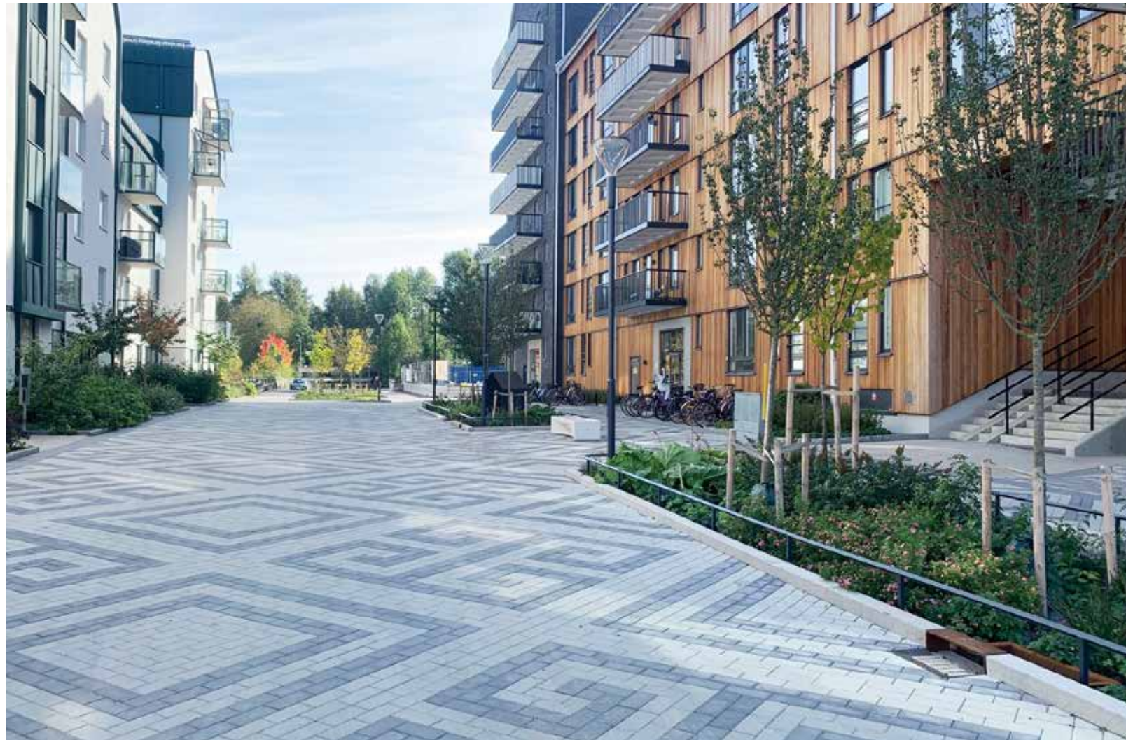
Amanuensgatan in Rosendal with an open subbase layer across the width of the street space with raingardens capturing runoff
